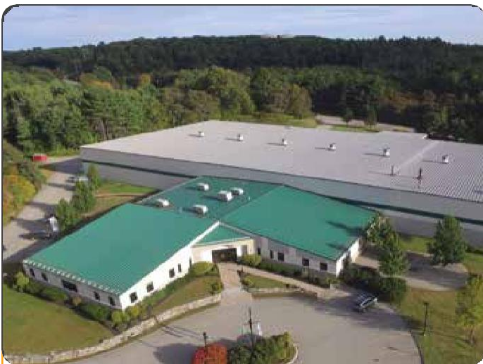
Modula Headquarters and Plant – Lewiston, Maine
