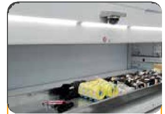
External Bay Lighting
