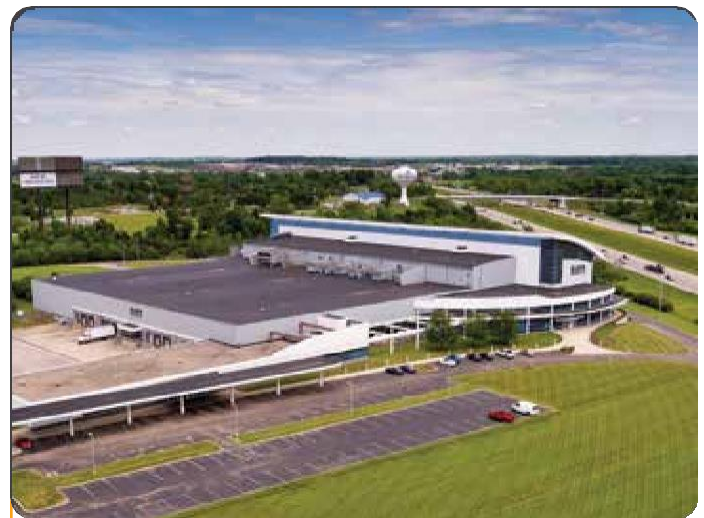
Modula Plant – Franklin, Ohio
